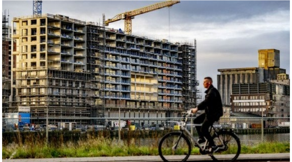
New homes under construction in Rotterdam, the Netherlands
